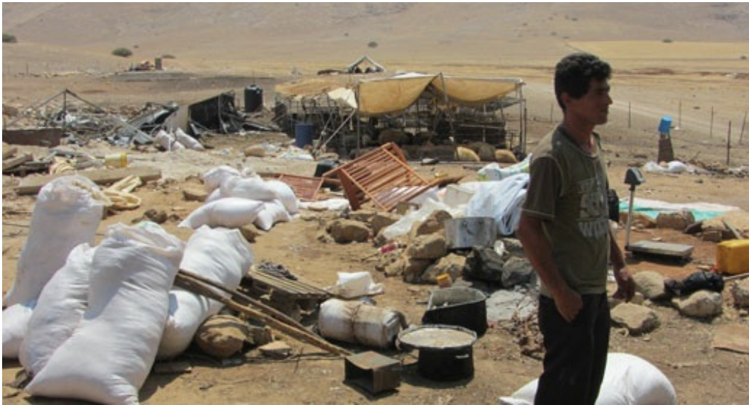
House demolitions in Khirbet Ras al-Ahmar, a community facing expulsion in the Jordan Valley. Photo: 'Atef Abu a-Rub, B'tselem, 30 July 2013
