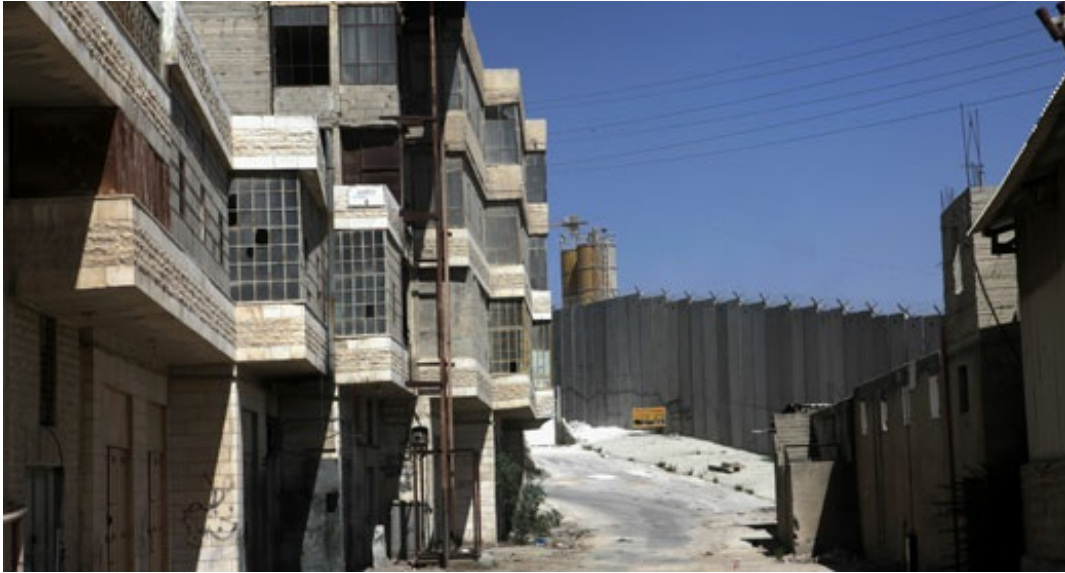
Abandoned buildings located near the Separation Barrier in the town of Bir Nabala, 24 September 2012. Photo: Anne Paq, activestills.org .
